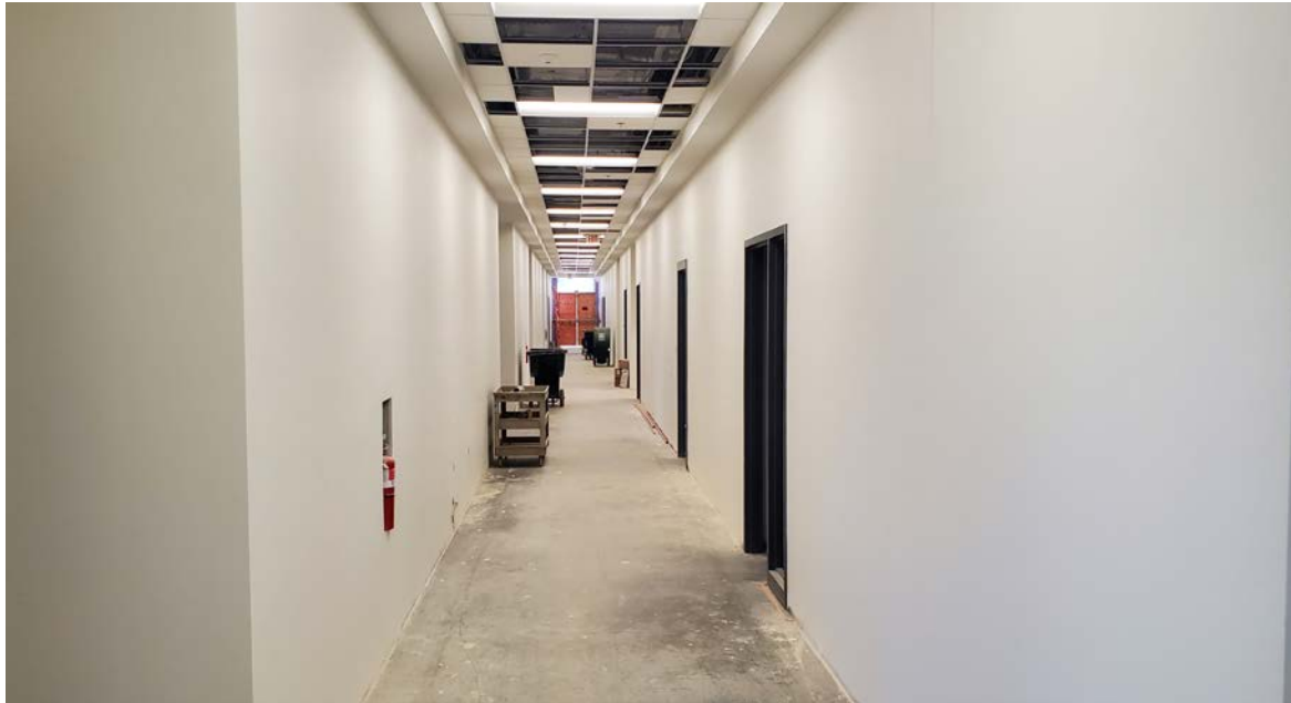
Classroom/Admin Bldg Main Hall February 2025
