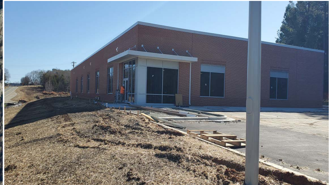
Classroom/Admin Building February 2025
