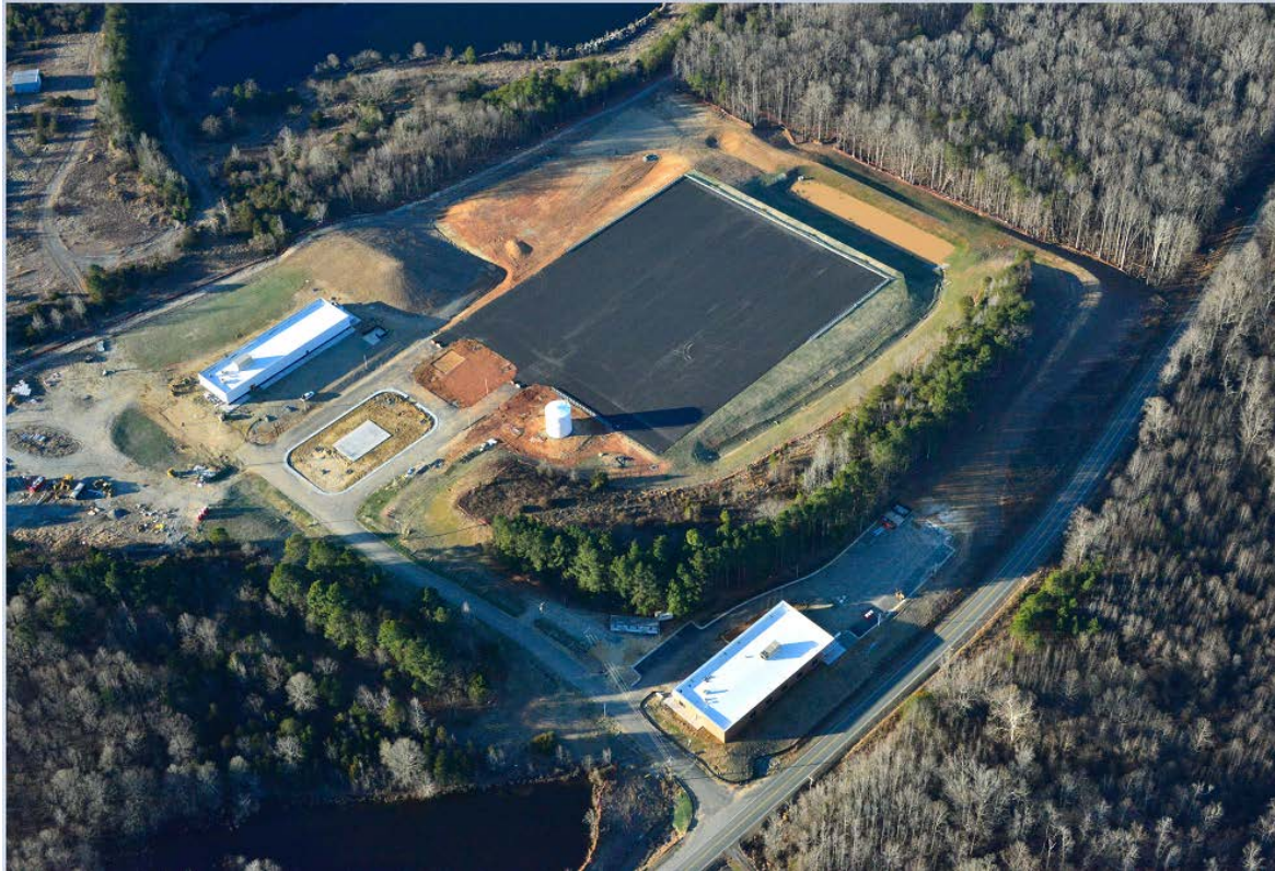
Overall Training Center Site January 2025
